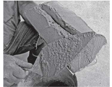
**B. Place Corner Stones First** — Alternate the long and short ends of each corner stone.
