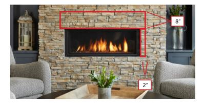
The area highlighted in red is a typical zone of risk related to excessive heat driven color change. Dimensions may vary slightly by manufacturer. Check with fireplace manufacturer to verify temperatures will not exceed 350° F.
