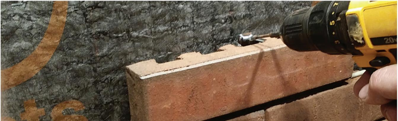
Our Dry-Stack mortarless option is a single 1-step installation. All you need is a brick, fastening clip, screw, butyl string, starter angle and rainscreen. With BRiKclad, you can begin enjoying your new clay brick wall in a matter of minutes!
