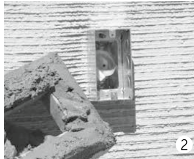
Apply mortar to back of Electrical Box Stone or prepared substrate.
